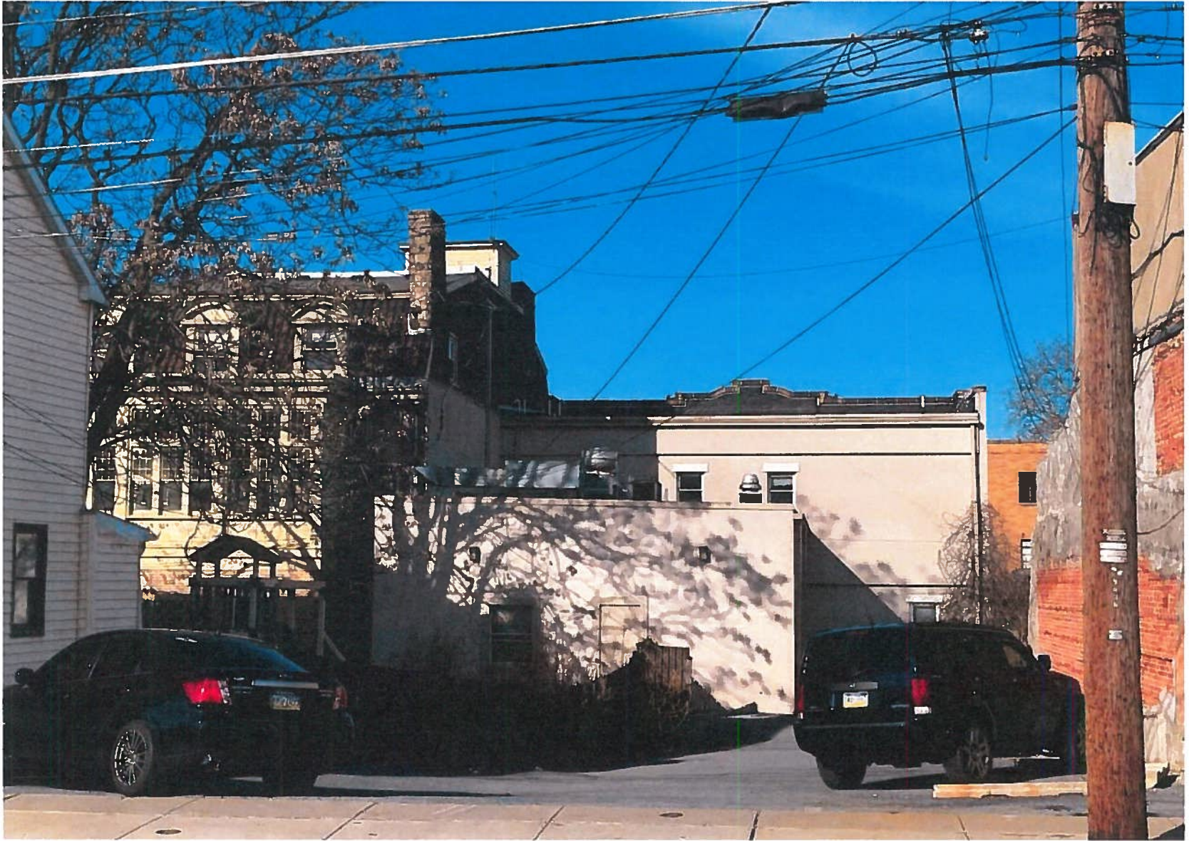
202-204 THIRD STREET & 206-208 THIRD STREET - Rear
