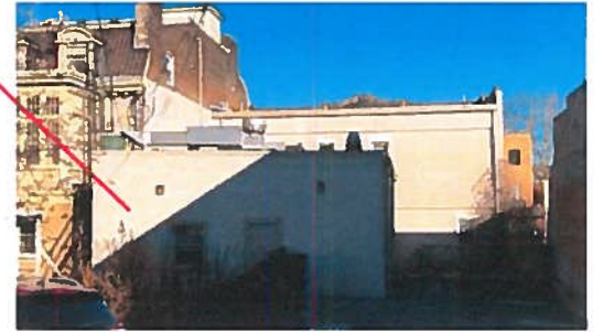
Rear (South) Facade of 206-208 Third Street
